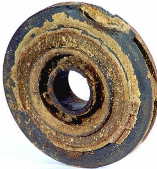
Fig. 1. Multiple faults and corrosion, caused by salt accumulation
